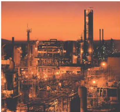
Industry and Building Automation
